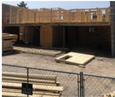
Framing of exterior walls and first and second floors is underway
