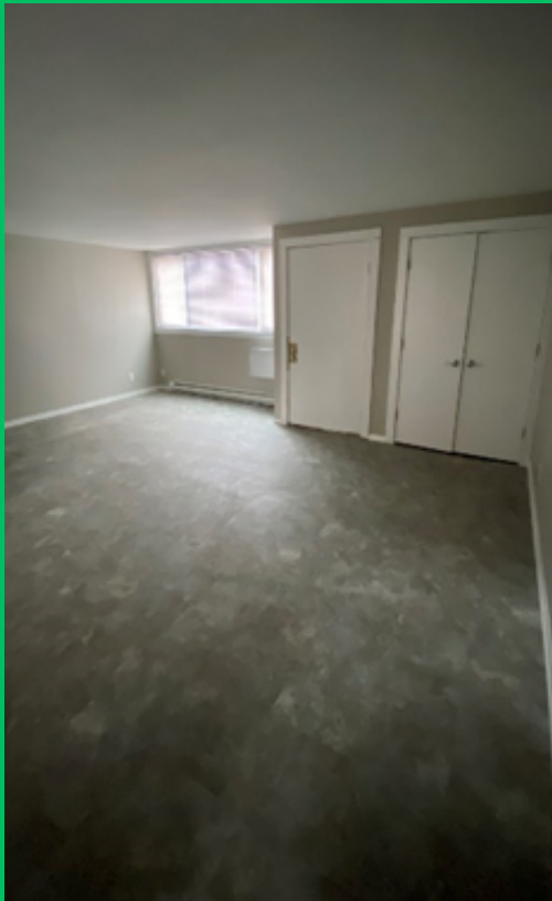
Photo of renovated living area.
