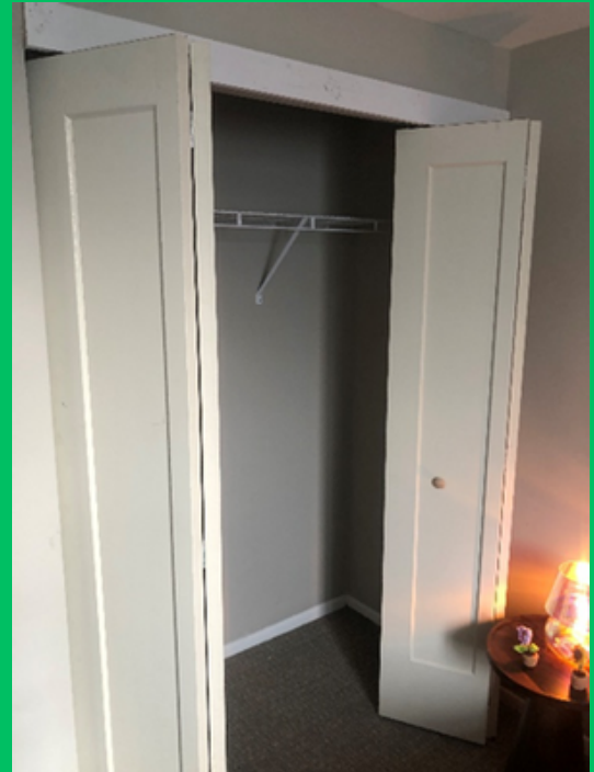
Photo of Renovated Closet.
