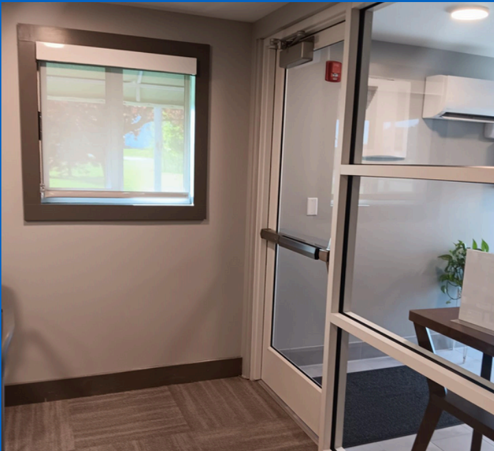
Photo of renovated leasing office conference room door.
