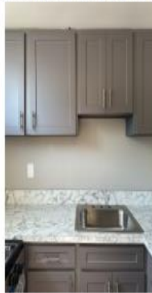
Newly Renovated Kitchen
