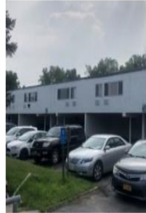
Exterior Painting is underway
